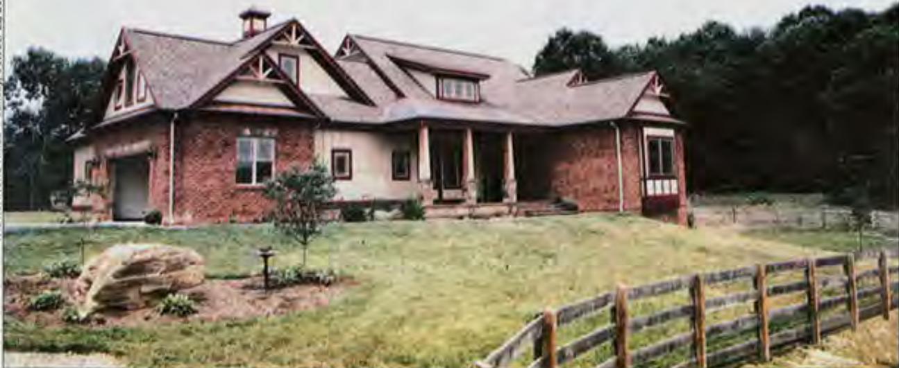
Jason Boyle, a partner in Green Valley Builders, built an EarthCraft-certified home for himself.
