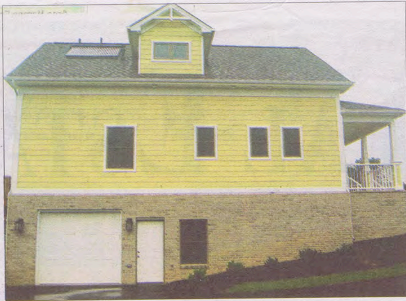
This occupied home (left) in Mount Tabor Meadows has a solar panel that heats the hot water, reducing the hot water bills by up to $40 per month. Pat Bixler (below) of Alt Energy stands in front of the solar hot water heater, which uses a back-up on-demand hot water heater on grey days.
